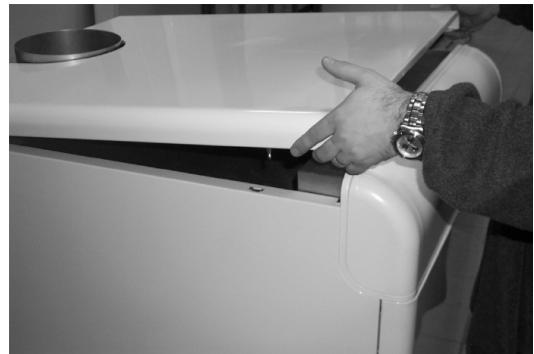
Fig. 4 - Lift by pressing upwards and take off the cover that is held at the sides of the boiler by pins.
